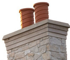
Appears open with clay or terra cotta liners
