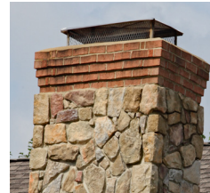
Appears closed by animal guard/ spark protector
