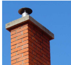
Appears closed by metal liner - may not be visible
