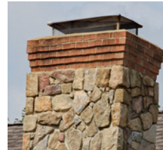
Appears closed by animal guard/ spark protector
